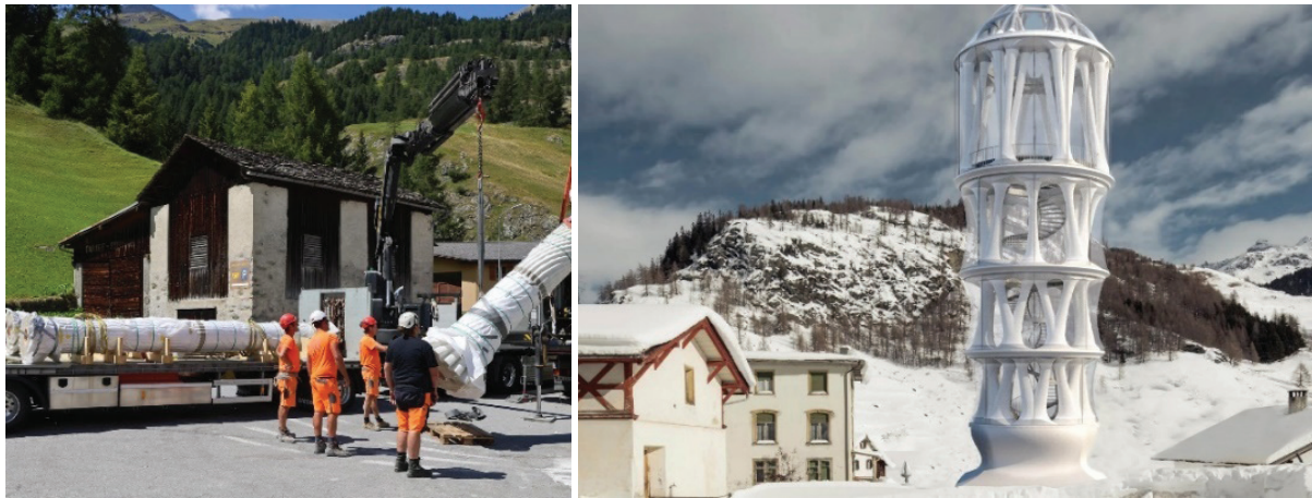
(B) Transportation and erection.
